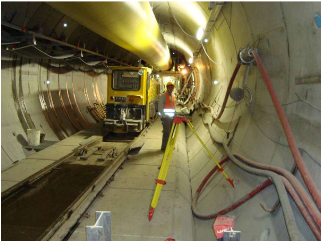
Controllo scavo meccanico TBM, Tunnel BBT
